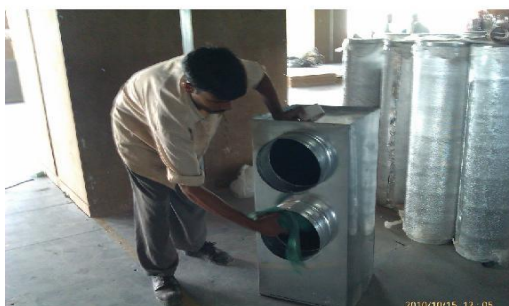
Ducts Wrapped With Plastic To Avoid Dust with Plastic Cleaning Prior To Installation
