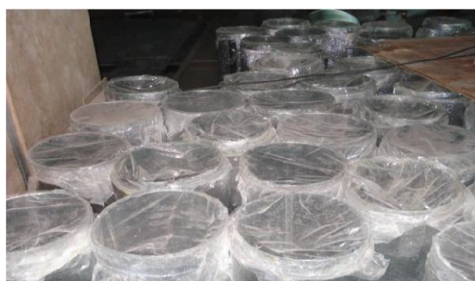
Ducts Stored with Properly Wrapped
