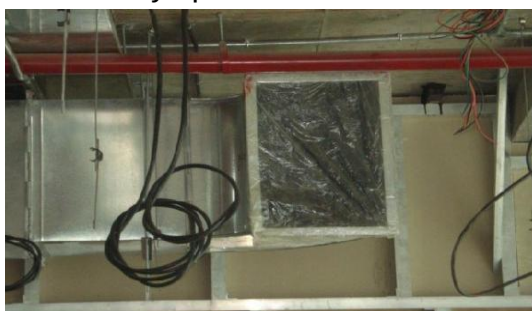
Ducts Wrapped With Plastic To Avoid Dust with Plastic Cleaning Prior To Installation
