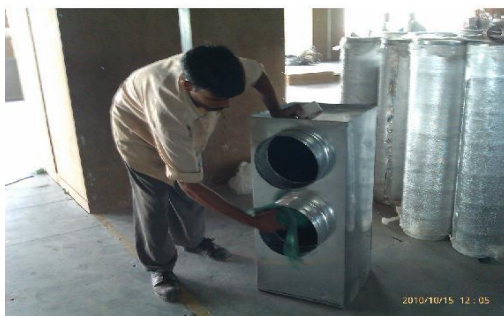
Cleaning Prior To Installation
