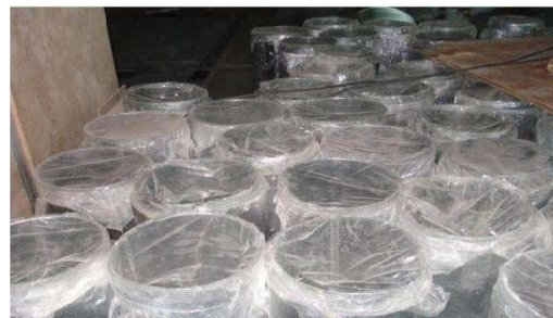
Ducts Stored with Properly Wrapped with Plastic
