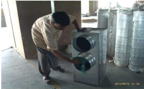
Cleaning Prior To Installation
