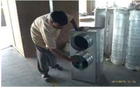
Cleaning Prior To Installation
