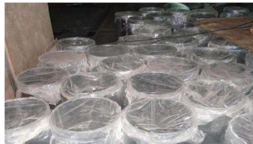
Ducts Stored with Properly Wrapped with Plastic
