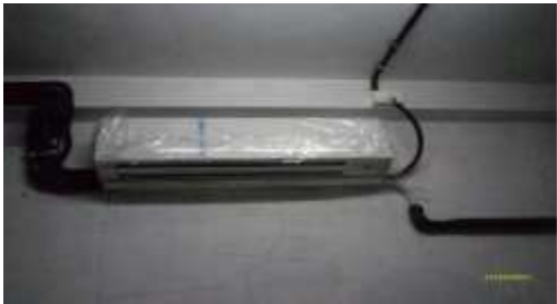
Equipment covered during Construction Phase
