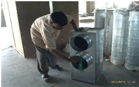
Cleaning Prior To Installation
