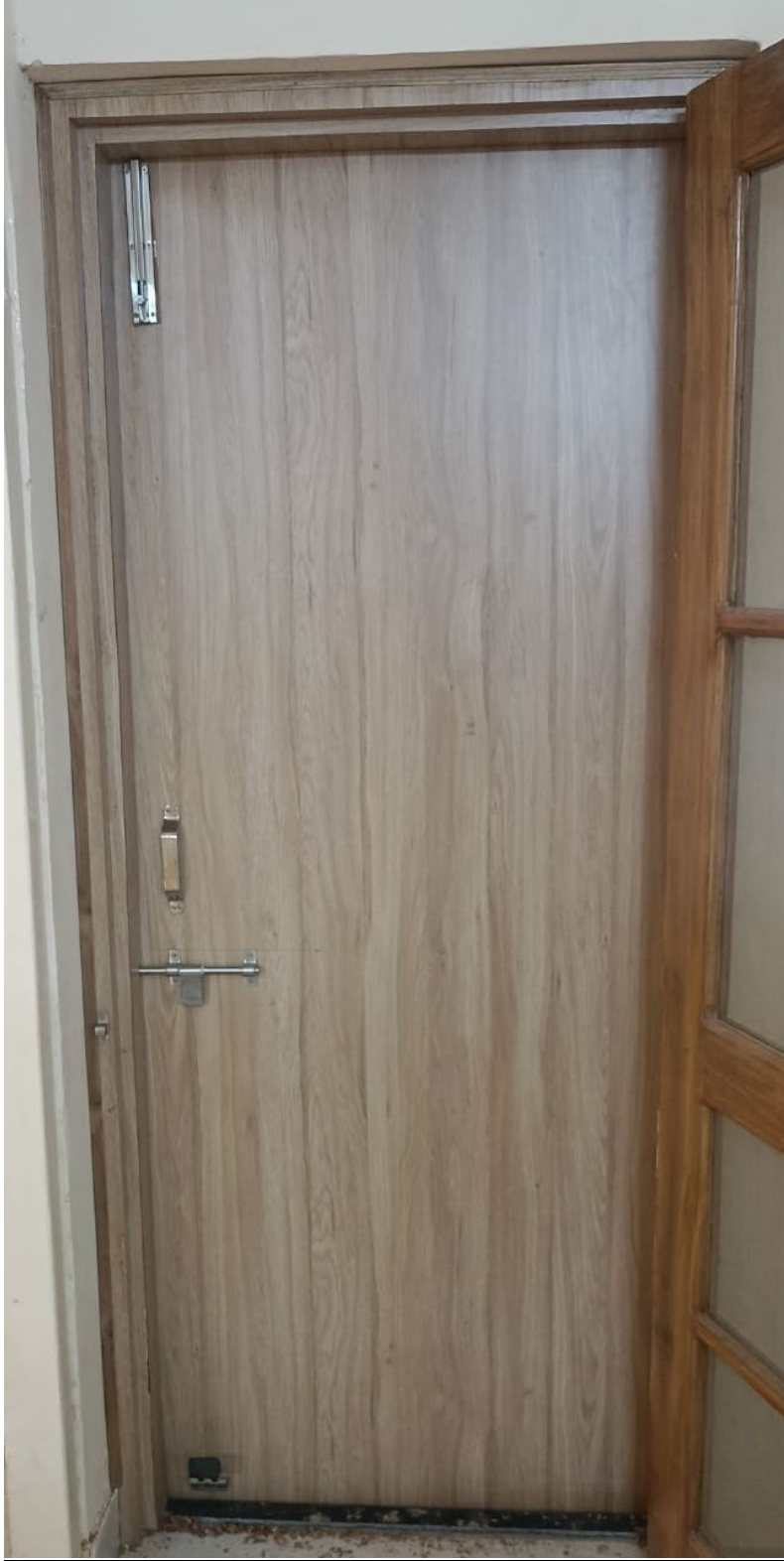
Inner side of Balcony gate
