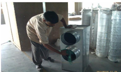
Ducts Wrapped With Plastic To Avoid Dust Cleaning Prior To Installation
