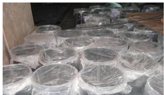
Ducts Stored with Properly Wrapped
