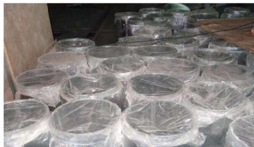
Ducts Stored with Properly Wrapped with
