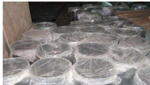
Ducts Stored with Properly Wrapped with Plastic
