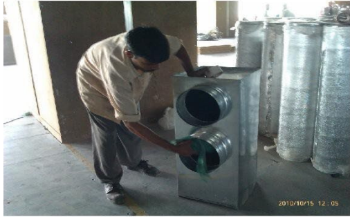
Cleaning Prior To Installation
