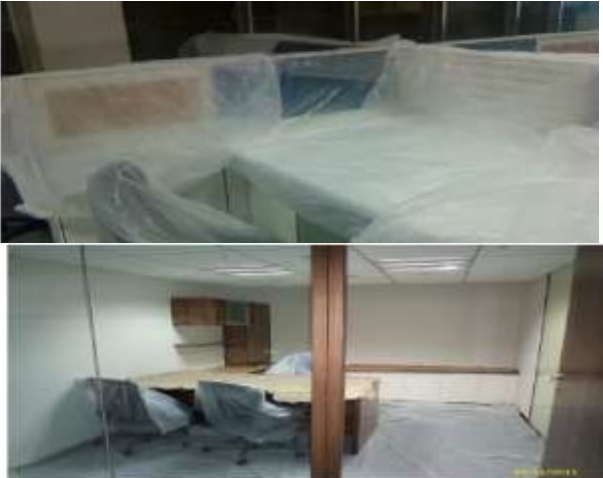
Equipment covered during Construction Phase
