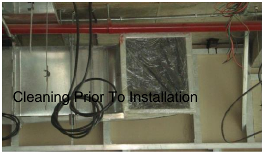
Ducts Wrapped With Plastic To Avoid Dust Ducts Stored with Properly Wrapped with Plastic
