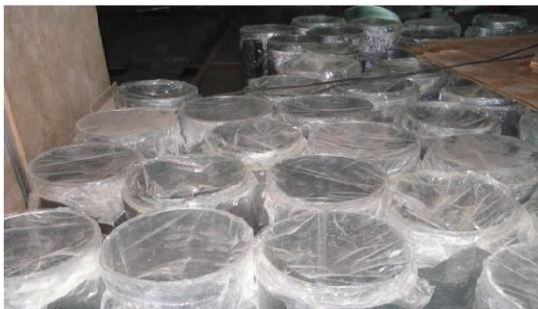
Ducts Wrapped With Plastic To Avoid Dust Ducts Stored with Properly Wrapped with Plastic
