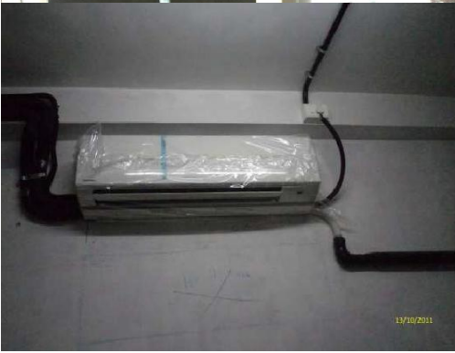
Equipment covered during Construction Phase Phase
