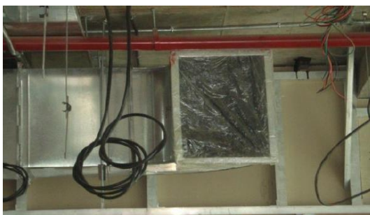
Ducts Wrapped With Plastic To Avoid Dust
