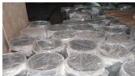
Ducts Stored with Properly Wrapped with Plastic
