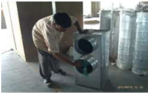
Cleaning Prior To Installation
